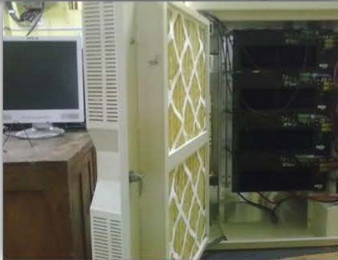
FUEL CELL SYSTEM (Back Up Source)
